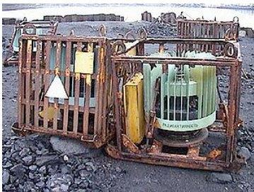
Soviet RTGs in dilapidated and vandalized condition, powered by Strontium-90 ^{90}\text{Sr} .
