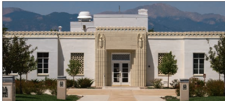
Peterson's museum was the original home of the Colorado Springs Municipal Airport Terminal.
